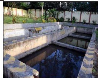
Clear water tank
