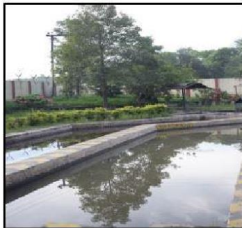
Primary settling tank
