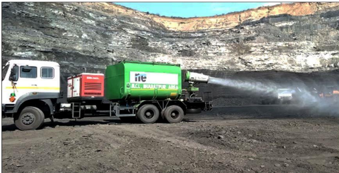
Truck Mounted Fog cannons for dust Suppression at Coal face area
